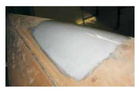
Photo 9—A mix of G/flex 650 and 503 Gray Pigment was applied as a sealer/undercoating and a bit of camouflage.
